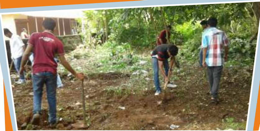
Volunteering Toilet Constructions for the Marginalised
